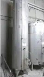
3.150 Liter storage tank
