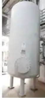
6.800 Liter Storage Tank / Pressure Tank
